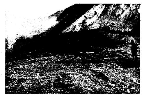
Figure G16. November, 1963. Two piezometric tubes observed on the Altopiano della Pozza bent by the return wave, which overran the area towards the south.
